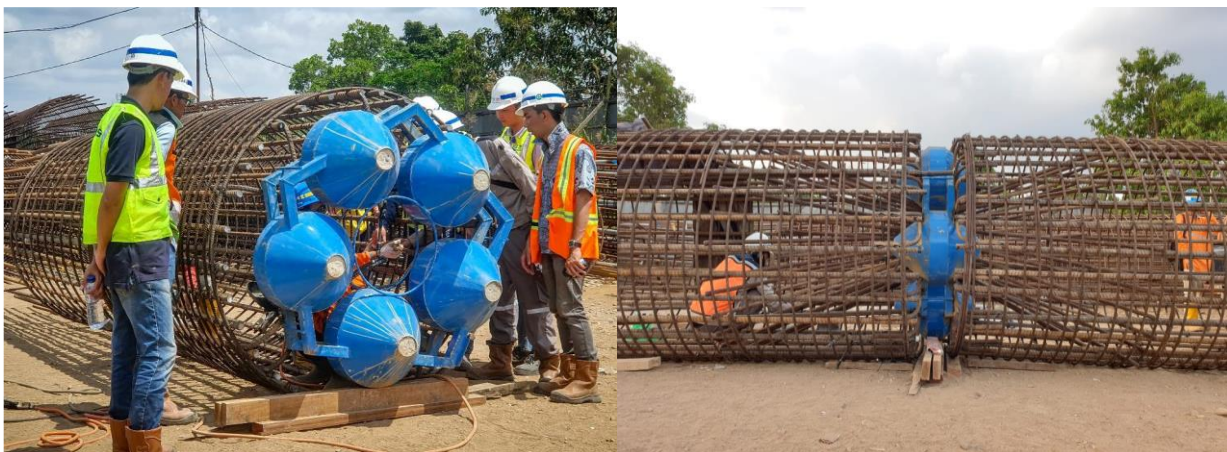
Fig 5. Bi-axial Osterberg Cell installation
