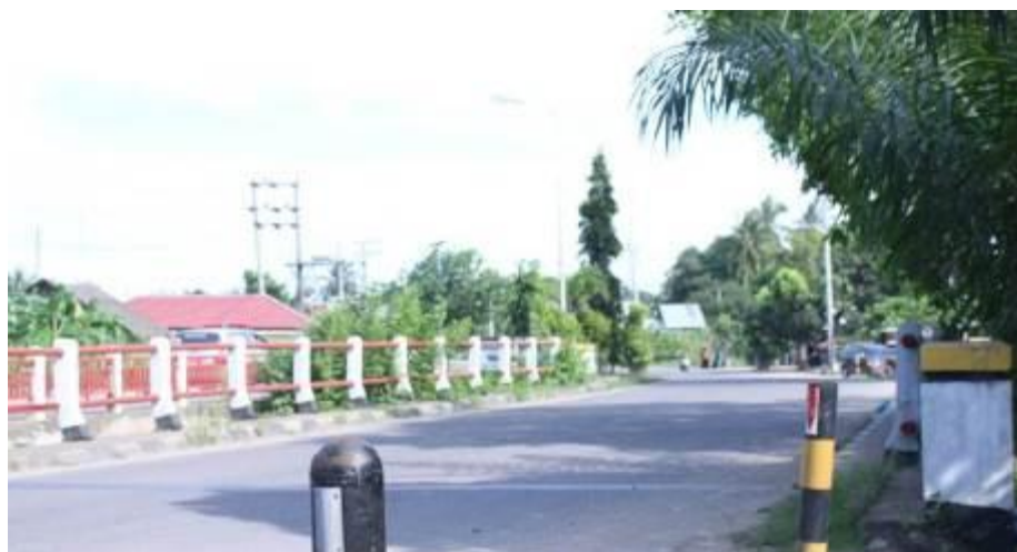
Fig 3. View of the Alue Raya Bridge
