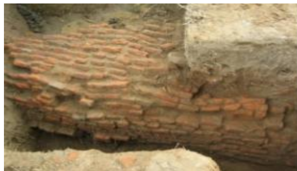
Fig 6. The brick structure around the Cot Astana site Source: Oetomo dan Surachman, 2012
